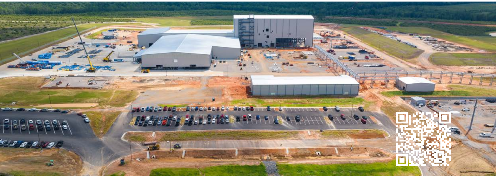
Aurubis Richmond, Georgia, USA – status as of August 2, 2023.
